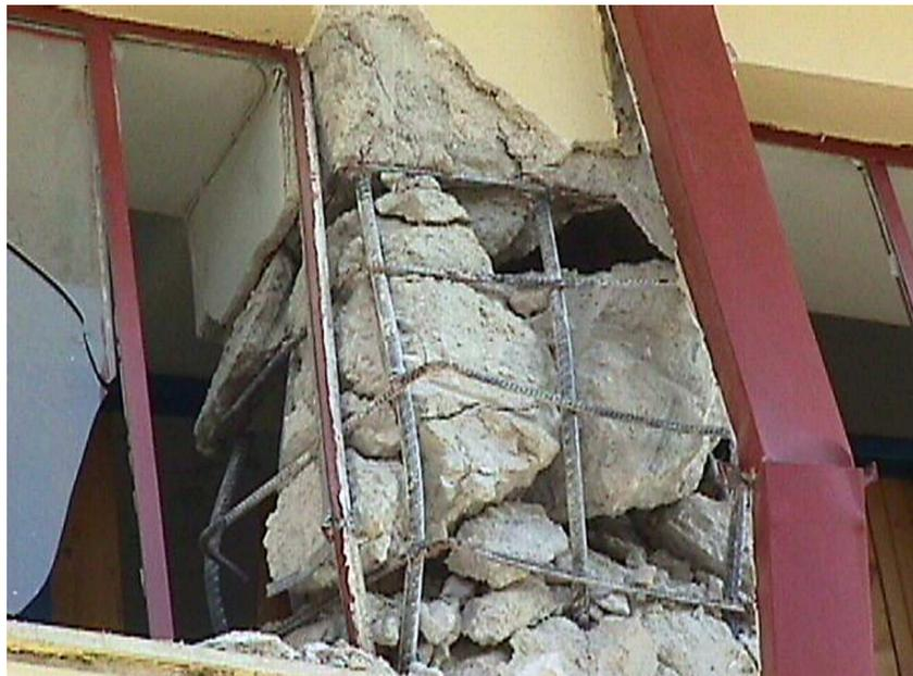
*Failure of a column dimensioned according to old regulations that required a peripheral stirrup with its end bent in  $90^\circ$  instead of  $135^\circ$  ( $45^\circ$ ).*
